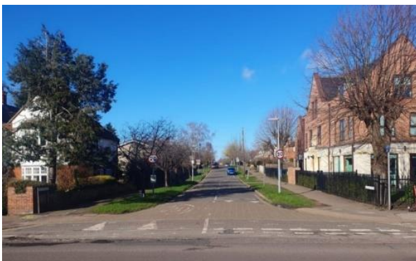
Left: Ascham Road / Milton Road junction where a new Copenhagen crossing will be constructed.
